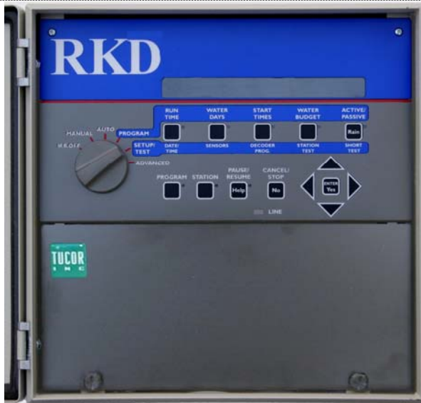
The RKD stand-alone 2-Wire controller supports from 1-100 valves
