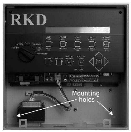
Figure 2.4. Marking up the mounting holes
